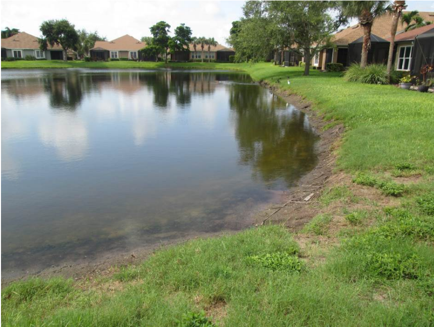
Pond 4 – 12” of vertical erosion along north and east bank, add plants
