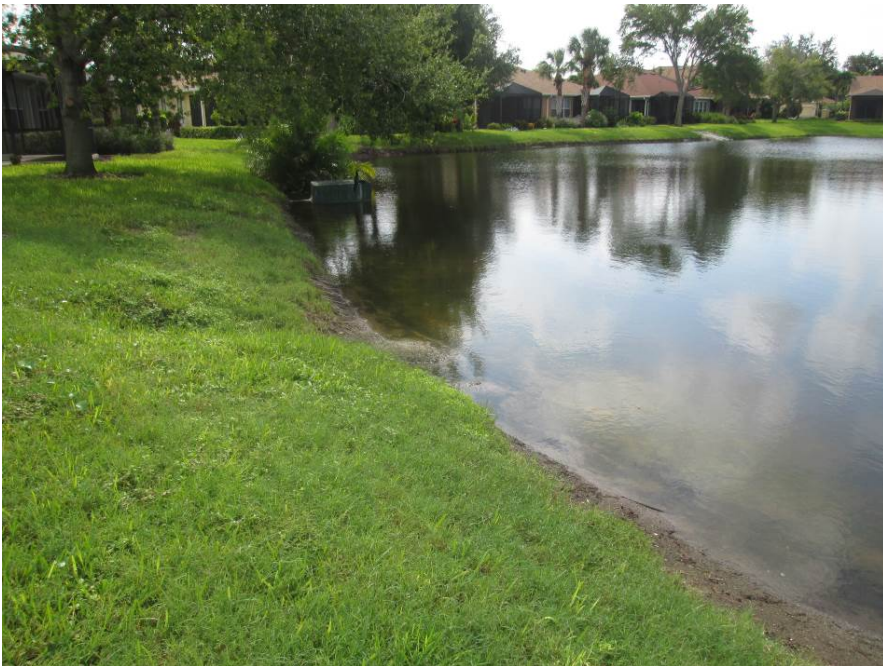
Pond 4 – Spot erosion on north side near west end
