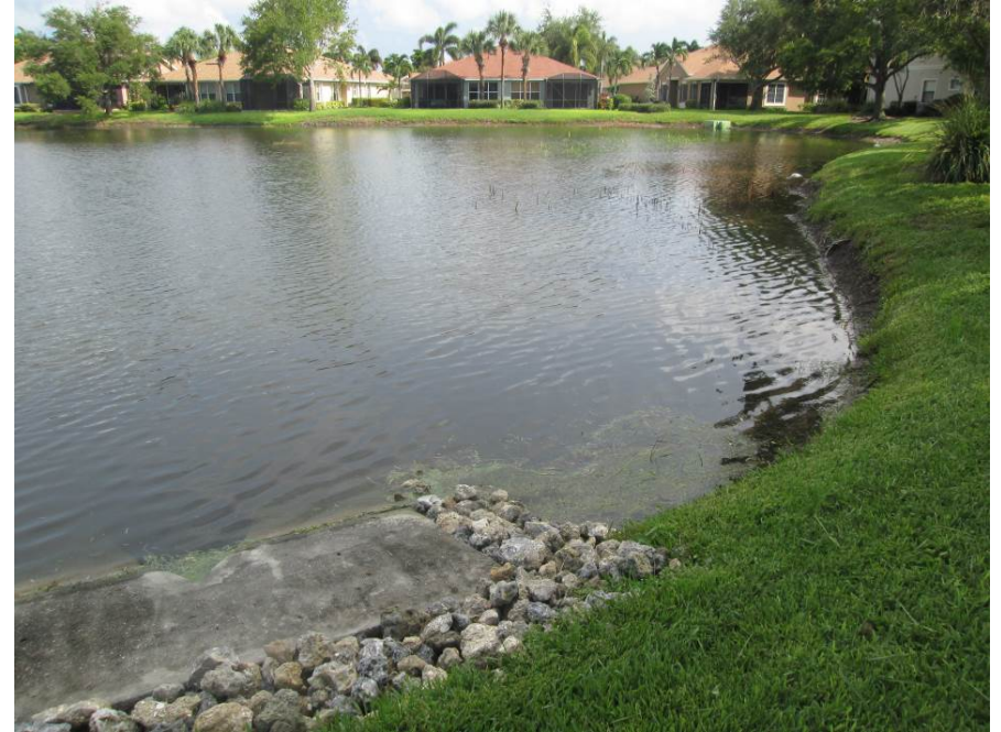
Pond 3 – 12"-18" of vertical erosion along east bank
