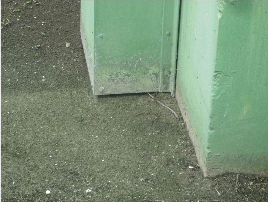
Pond 8 – Excavate 4”-6” under skimmer of control structure on west bank
