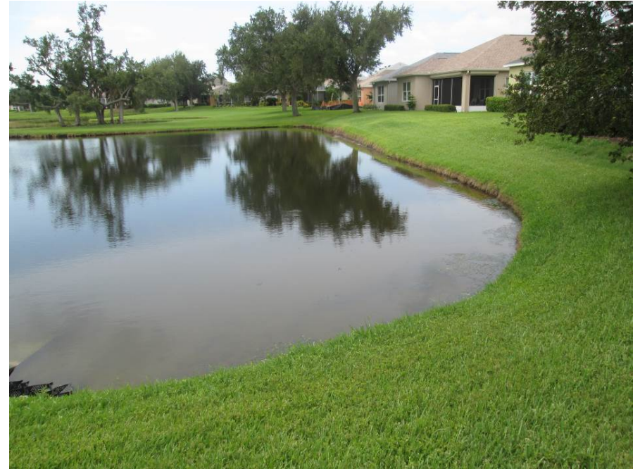
Pond 9 – 12” vertical erosion on west side near north bank
